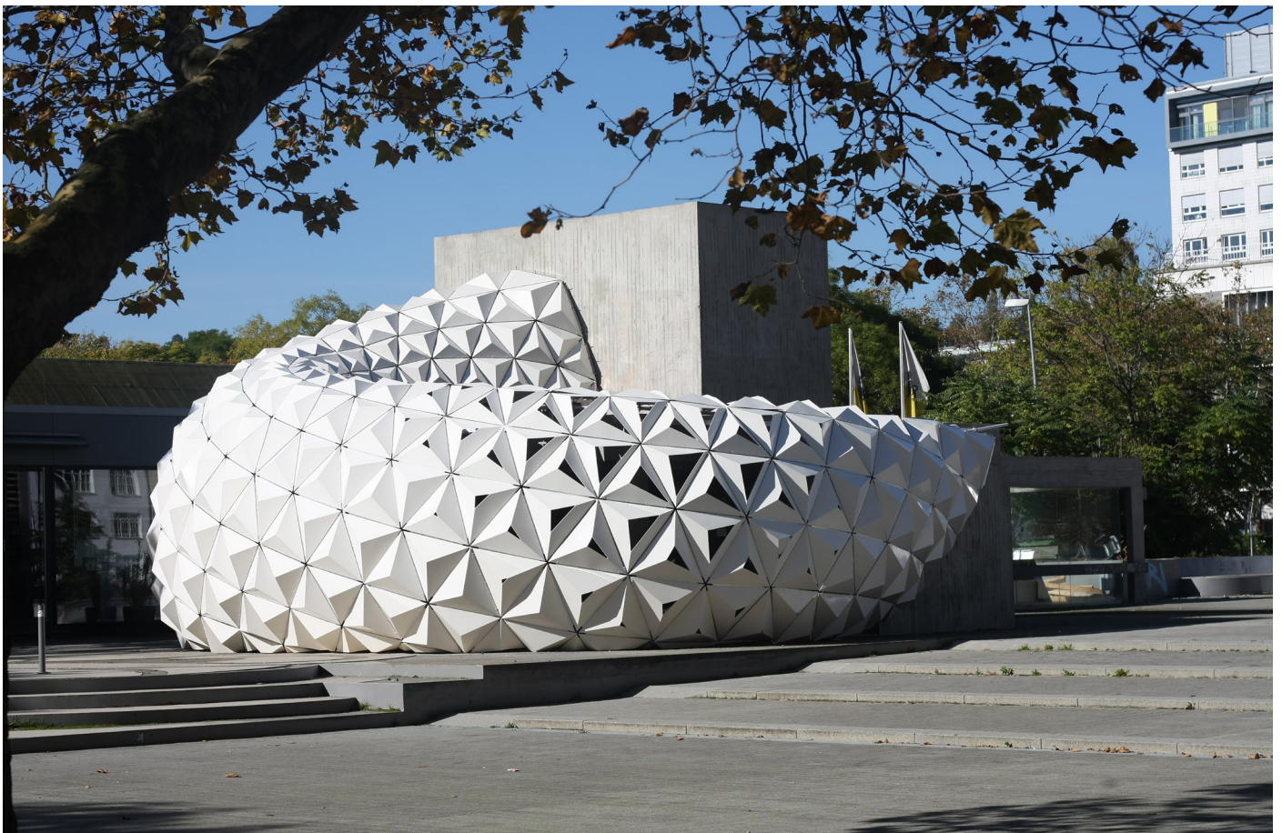
Figure 3: Arboskin Building The ArboSkin pavilion at the University of Stuttgart is made from 388 biodegradable bioplastic panels. (Permission of Manfred Hammer)
